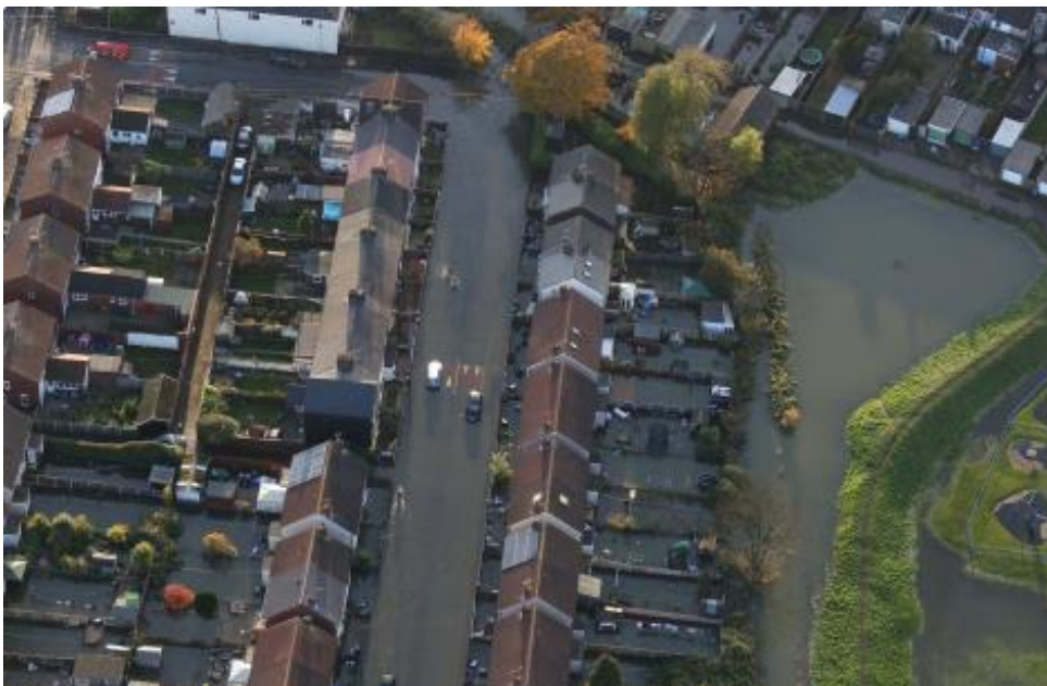
Figure 8. Flooding at Bentley during the 2019 flood event.
