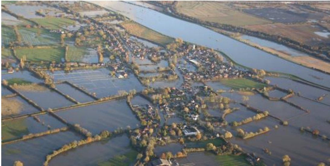
Figure 7. Flooding at Fishlake during the 2019 flood event.
